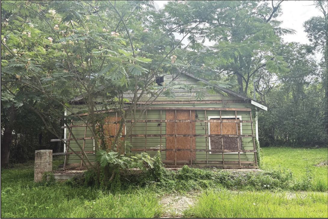
Dilapidated houses are common in Dewey City, a historic Black neighborhood in Thomasville. Many residents don’t have the funds to mitigate issues with mold, asbestos, or lead paint. (Briah Lumpkins/KFF Health News)
