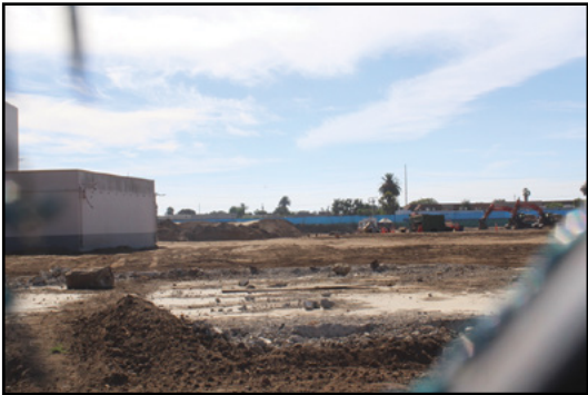
A photo of Inglewood High School under construction. (Photo by Marion Apio)
